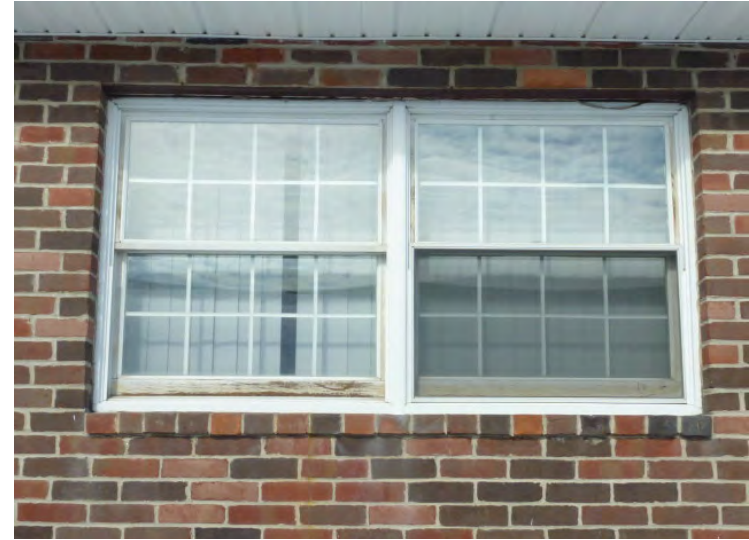
Windows are the originals and are 41 years old. Worn finishes, failing glazing gaskets, failing caulking and rusting steel lintels are all typical.
