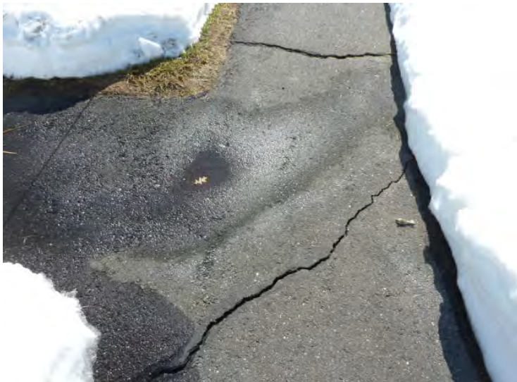
Typical asphalt walkway paving cracking and sub-base failure.
