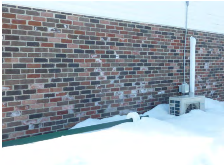
Efflorescence at select brick walls indicates historic moisture migration through the walls. The brick is shown to be cleaned mid-term.
