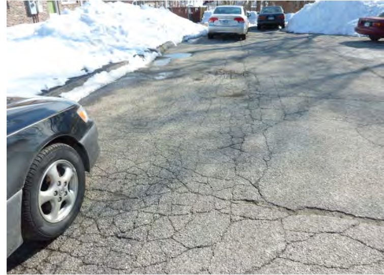
Typical asphalt drives paving sub-base failure.
